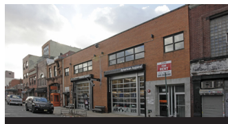
102 N 6th St | Williamsburg
