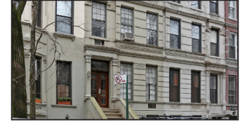
18 W 125 th St | Upper West Side
