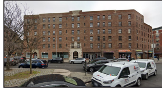
2802 Fredrick Douglass Blvd | Harlem
